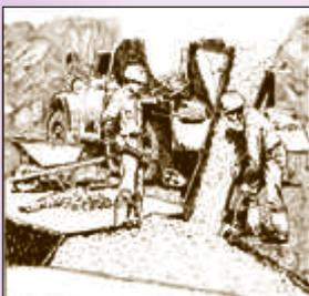
short-handled, square-end shovel is an effective tool for spreading concrete, but special concrete rakes or come-alongs also can be used. Excessive horizontal movement of the concrete not only requires extra effort, but may also lead to segregation of the concrete ingredients.
